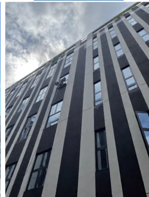
Stone + glass curtain wall
